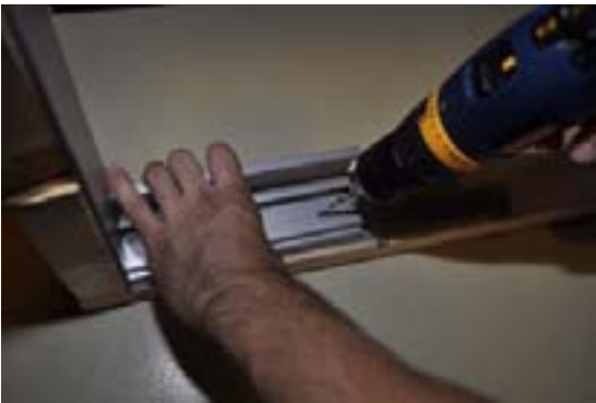
3) Drill holes for size and the number of screws to be used. This depends on frame type and wind load. 12" on-center is common.
