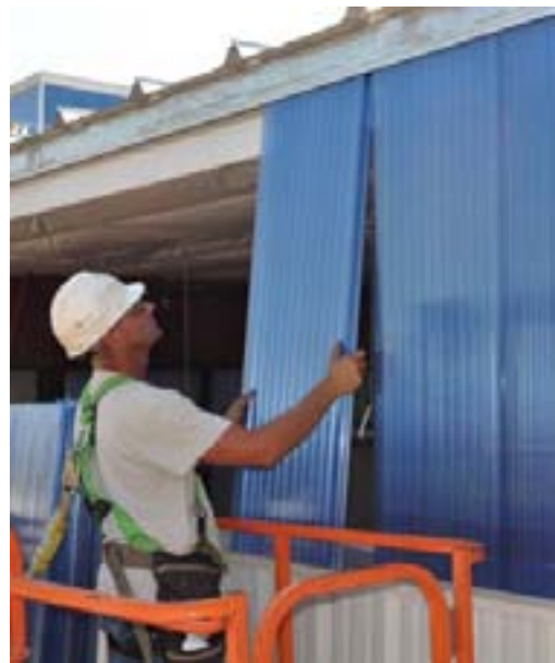
1) Insert the panels into the top profile (“U”). Tilt the panels just enough to allow it to get into the “U” profile
